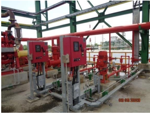
Electric Motor Driven Jockey Pumps
