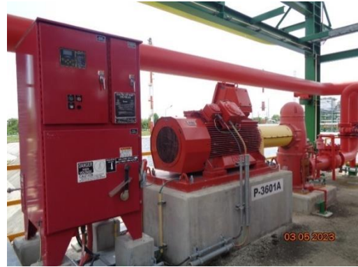
Electrical Driven Fire Water Pump
